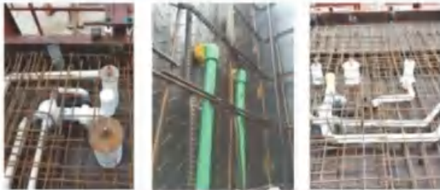
Installation of MEP and other cast-in items
