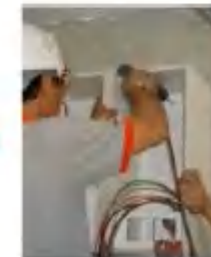
Install bracket for basin cabinet
