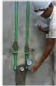
MEP works & Pressure test
