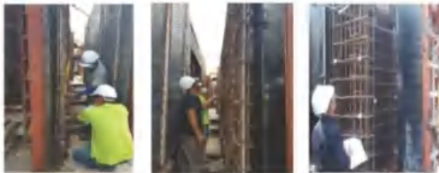
Inspection prior to concreting
